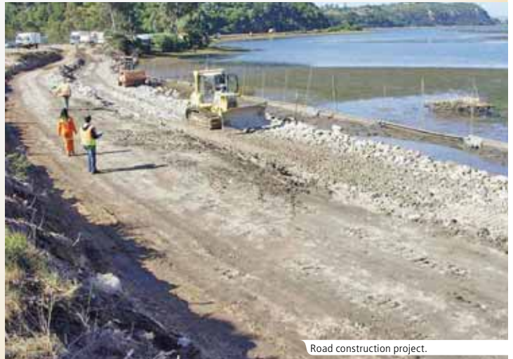
Road construction project.
